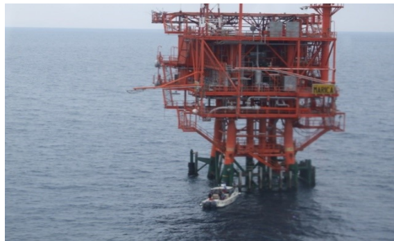
Figure 8. Gas platform Marica
